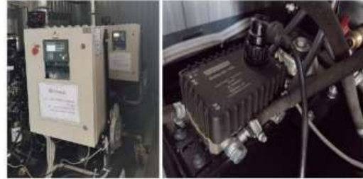
Fig. 6. Experimental energy complex equipment: diesel generators (left) and fuel flow meter (right).
